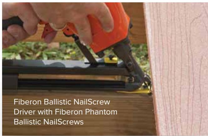
Fiberon Ballistic NailScrew Driver with Fiberon Phantom Ballistic NailScrews
